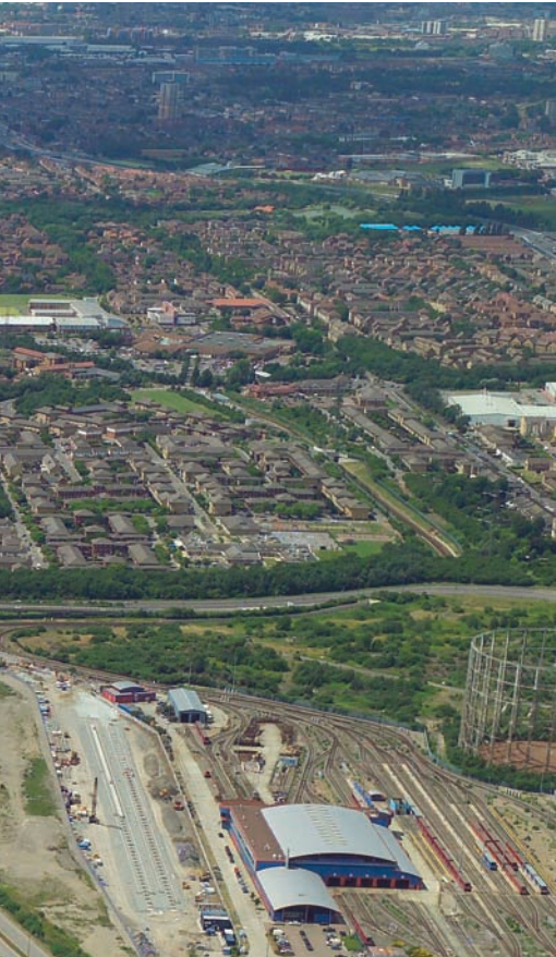
◀ Aerial view of Docklands, featuring the UEL campus, London City Airport, the ExCel Exhibition Centre and the O2 Arena
